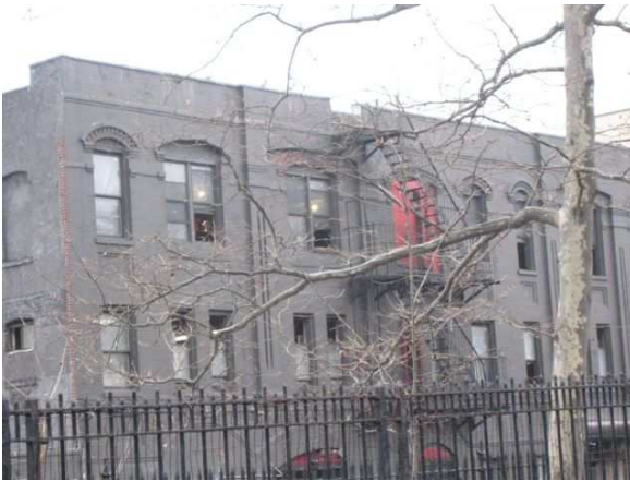
Upper two floors of Clinton Park Stables
